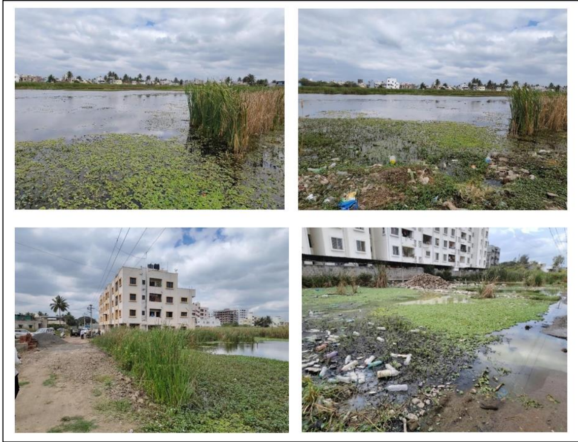
Figure 3 Stagnation of water in Gangotri Colony in Shamraonagar due to absence of proper storm water drainage system
